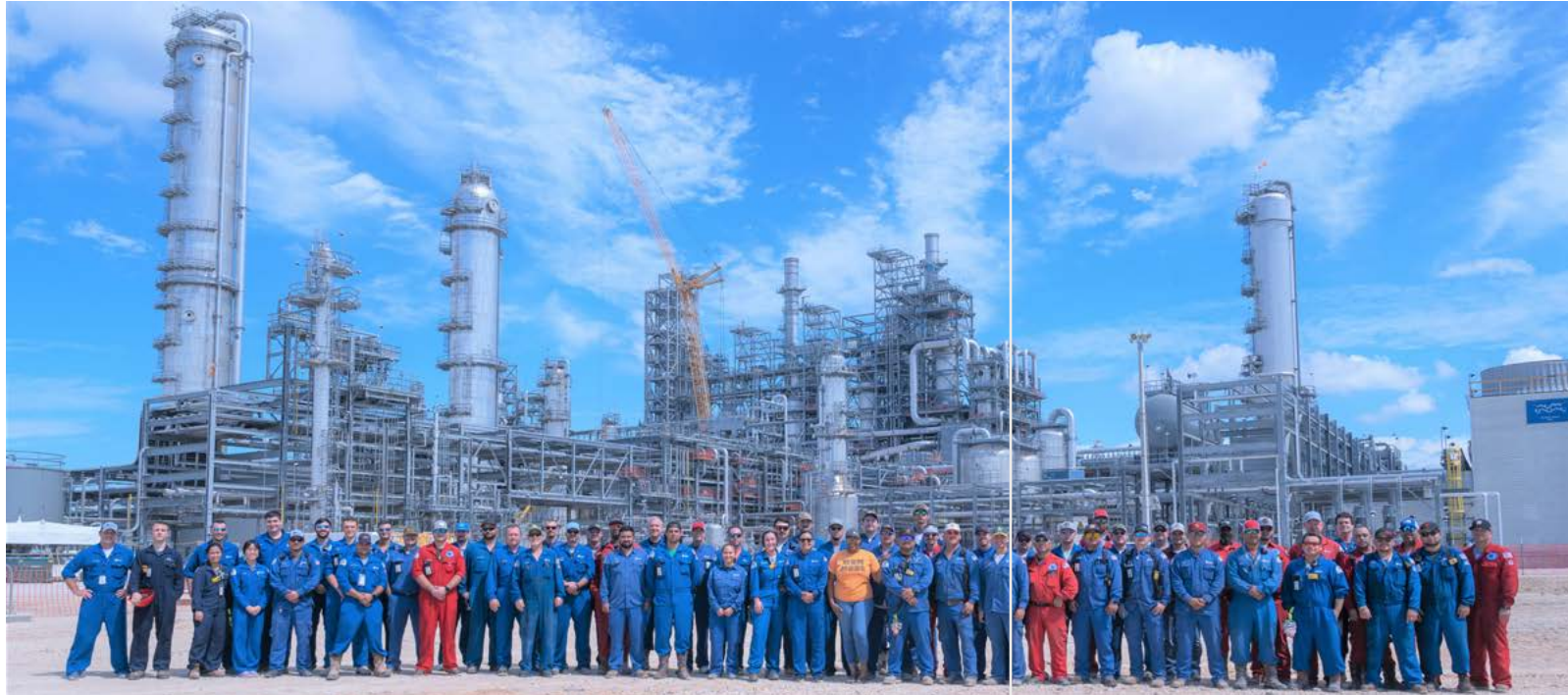
▲ Employees of Enterprise at its recently completed PDH 2 plant in Chambers County, Texas. Combined with Enterprise’s existing PDH 1 plant, the company can produce 3.3 billion pounds per year of polymer grade propylene (“PGP”) at its Chambers County, Texas complex. PDH 2 was modified from its original design to consume hydrogen produced as a by-product to reduce CO 2 emissions.
